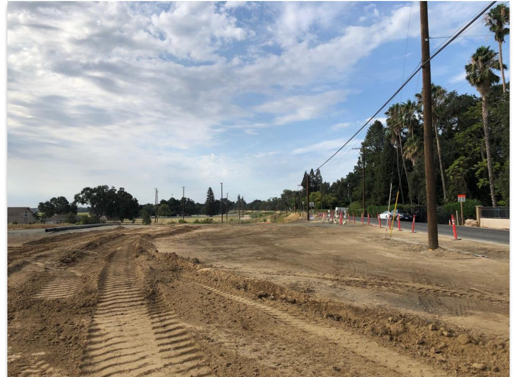
Reach A Overhead Utility Relocations, Site Preparations, 2022
